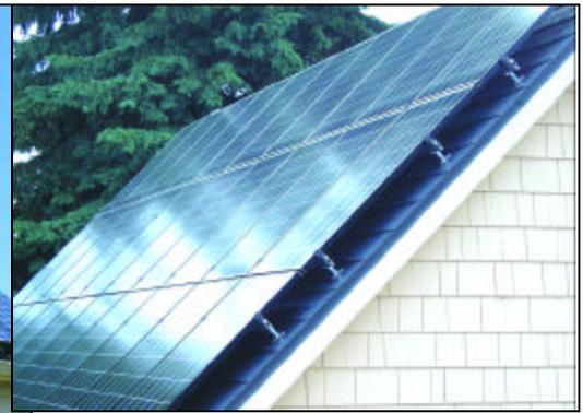
By happy coincidence, the 45-degree angle and direction Eva's garage roof faces was nearly perfect for maximum PV power conversion.
